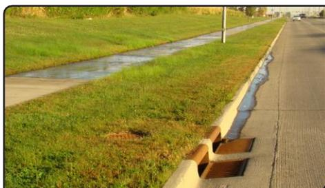
Rain water oozing under recently planted turf due to poor topsoil quality and compaction.
